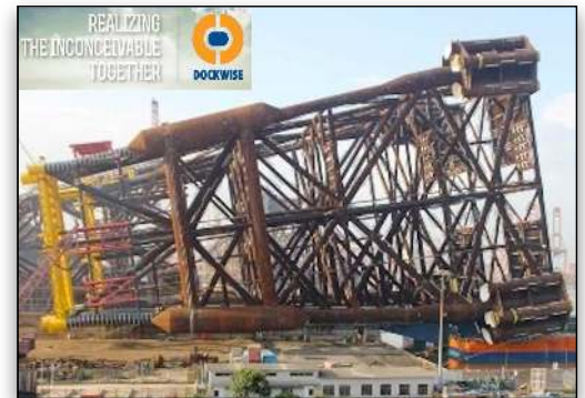
SHWE Jacket Load-out.
