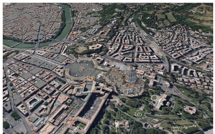
By working in a collaborative digital environment, Italferr saved 50 hours in modeling time, delivering the model 20 days ahead of schedule.
