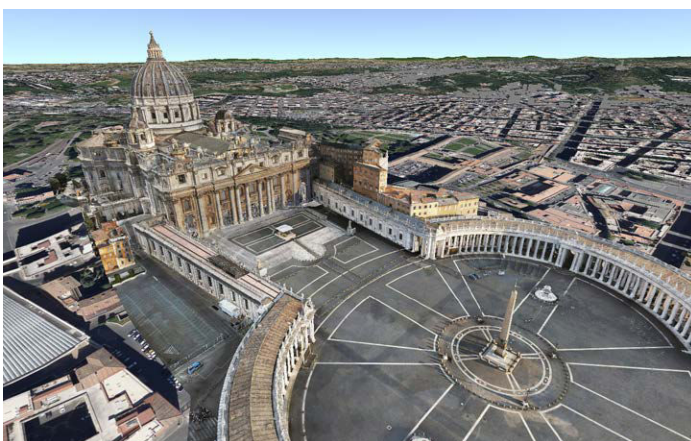
The Fabric of Saint Peter hired Italferr to create a digital twin of the structure.
