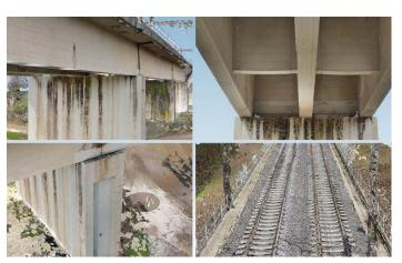
The Borratino viaduct is 1,300 meters long and made of reinforced concrete with 50 spans, making it difficult to efficiently integrate the data from several different technologies in sufficient detail.
