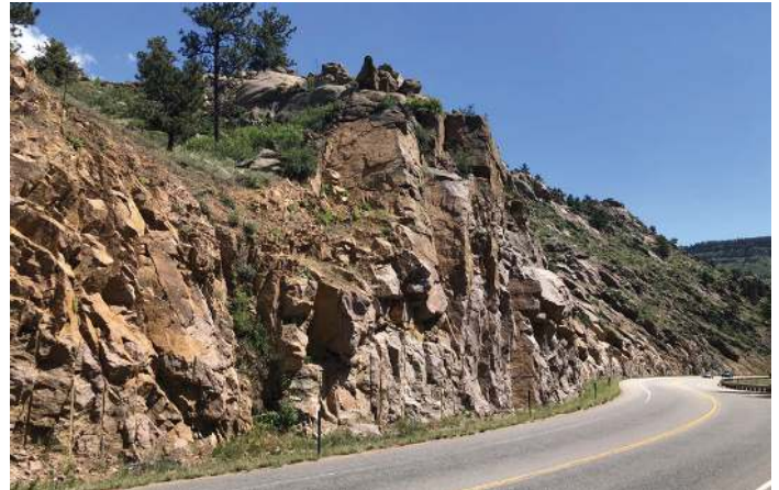
Data from the sensors provide a longer-term picture to understand ground and rock movements, helping prevent damage and ensure safety. Image courtesy of Shannon & Wilson.
