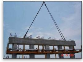
Precast reinforced concrete caps designed with LEAP RC-PIER were used for the majority of the spans.
