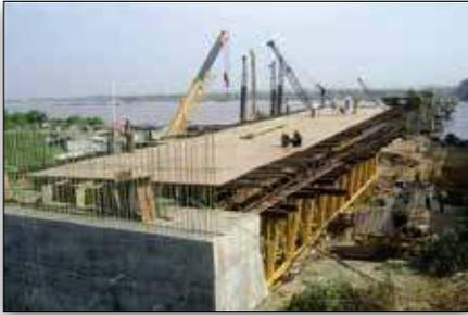
Figure 1: Superstructure Formwork Preparation
